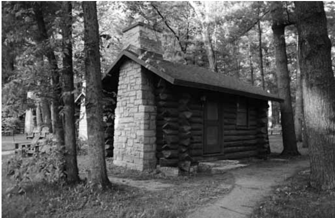
The lodge and cabins at White Pines Forest State Park in Mt. Morris were constructed by the CCC. Photo copyright IL Department of Natural Resources.
